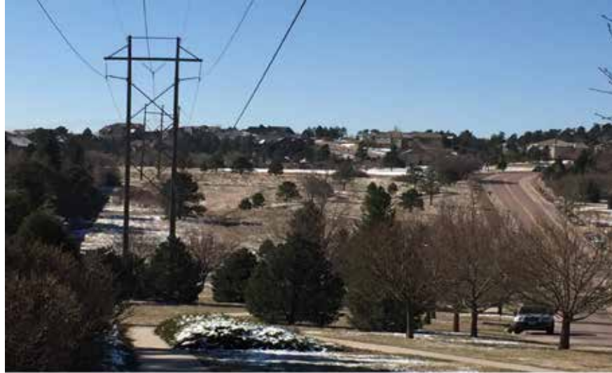
Colorado Springs overhead transmission line with underground distribution
