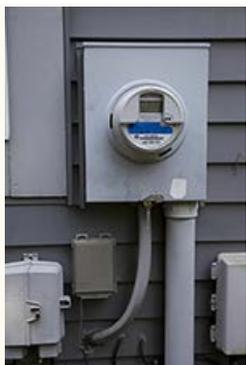
The heart of the Demonstration Project is the smart meter, a digital electric meter equipped with two-way communications technology.
