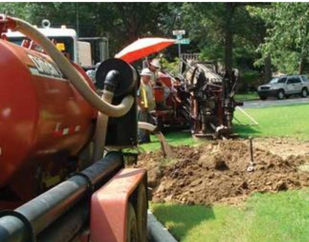
*Directional boring equipment is used to get the cable underground.*
