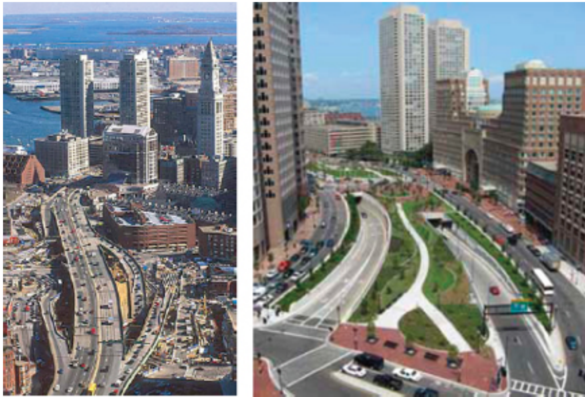
FIGURE 5.2 Boston Central Artery as an elevated structure and as an underground roadway SOURCE: MADOT, 2012.
