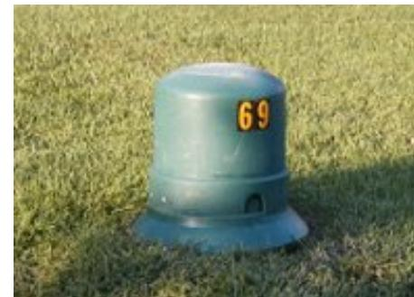
Because of their small size and weight, service pedestals do not have to be located close to streets or "improved" surfaces as padmount transformers do. Generally, a service pedestal needs to be located within 5 to 10 feet of the pole that has the overhead connections being undergrounded.
