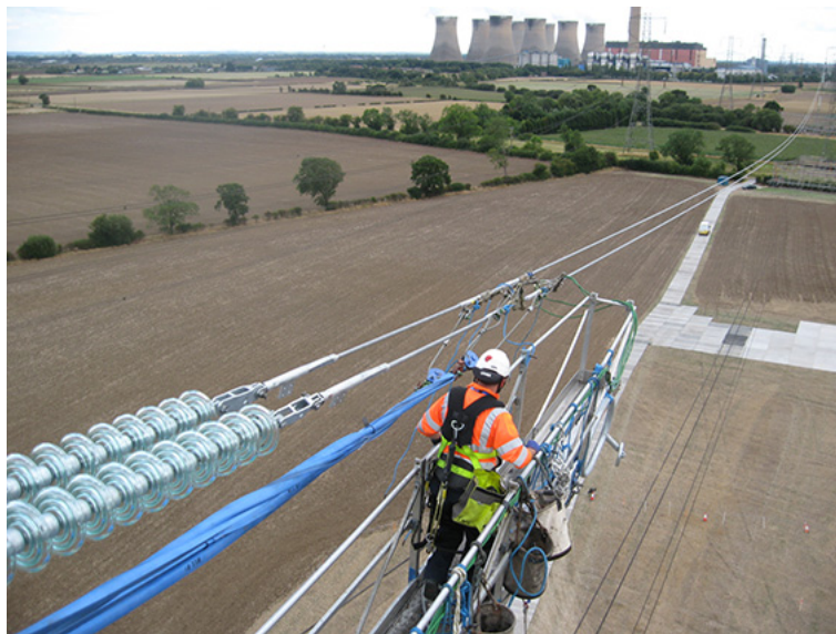
Power plant upgrade
