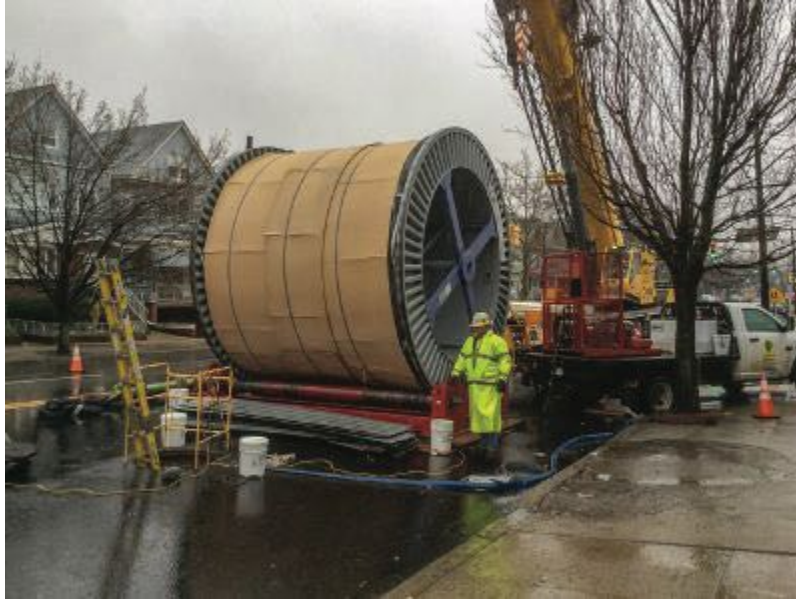
21 st Century undergrounding has come of age
