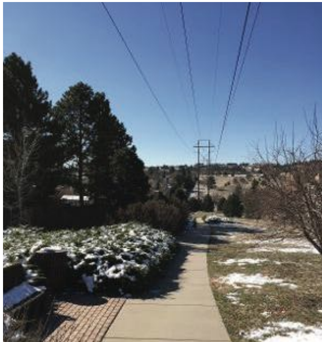
Colorado Springs overhead transmission line with underground distribution
