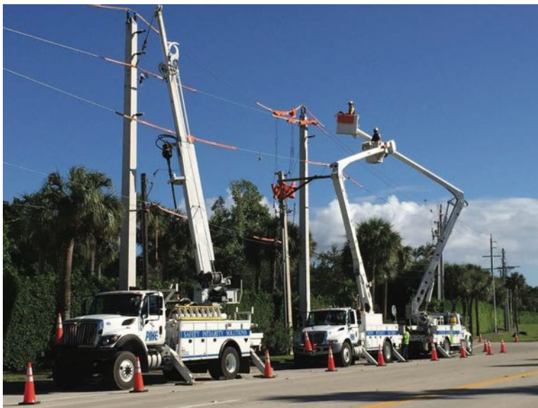
FPL contract crews at work hardening overhead lines
